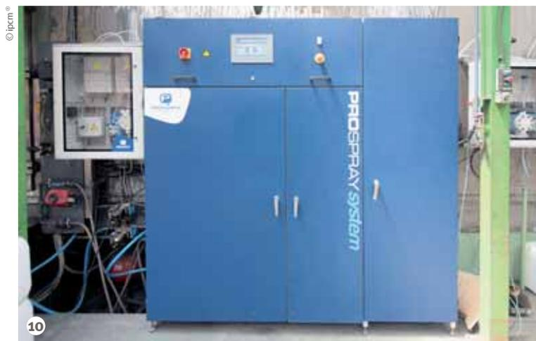
**Figure 10: Proquimia's Prospray atomisation system for the last passivation stage.**
